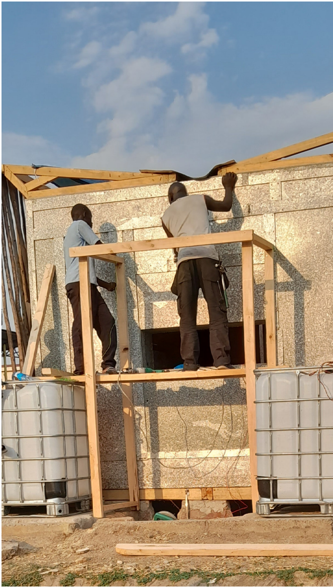
Figure 62. Assembly of the insulation walls and the solar PV panels and the water gutter on the roof
