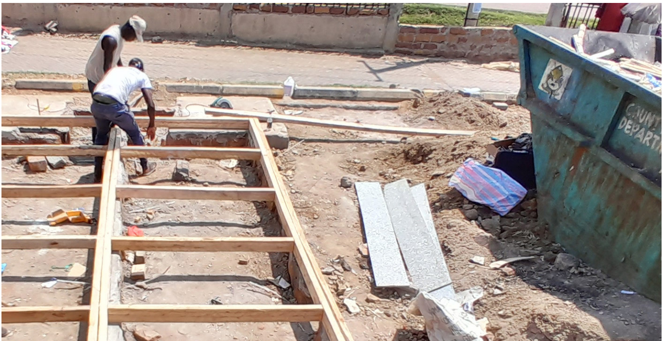
Figure 61. Construction of the low-carbon cold room foundations and insulation walls
