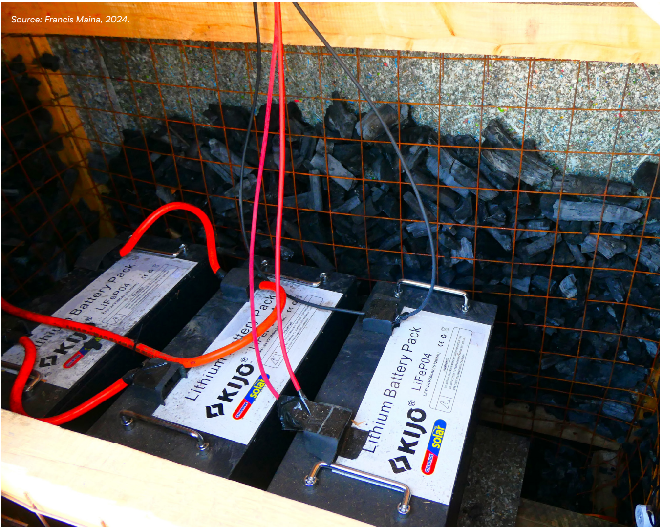
Figure 38. Installation of the charcoal inside the technical room
