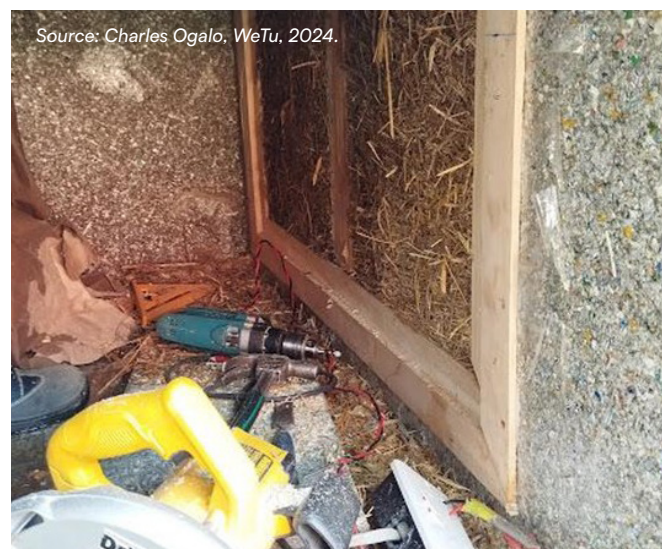
Figure 19. Replacement of eco-boards with T&G timber to protect straw bale from high humidity
