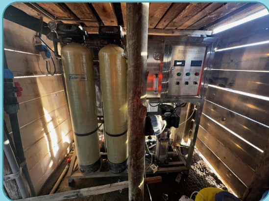
Water filtration unit rejects 50% of water as unfit water for consumption.
