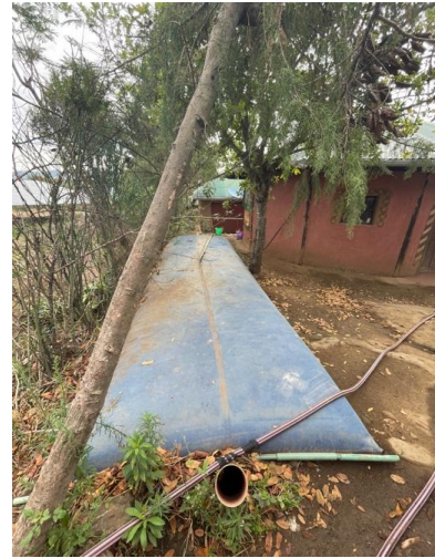
Image 20D: Biogas flex tube trialling use of opuntia pads mixed with cow dung for biogas generation
