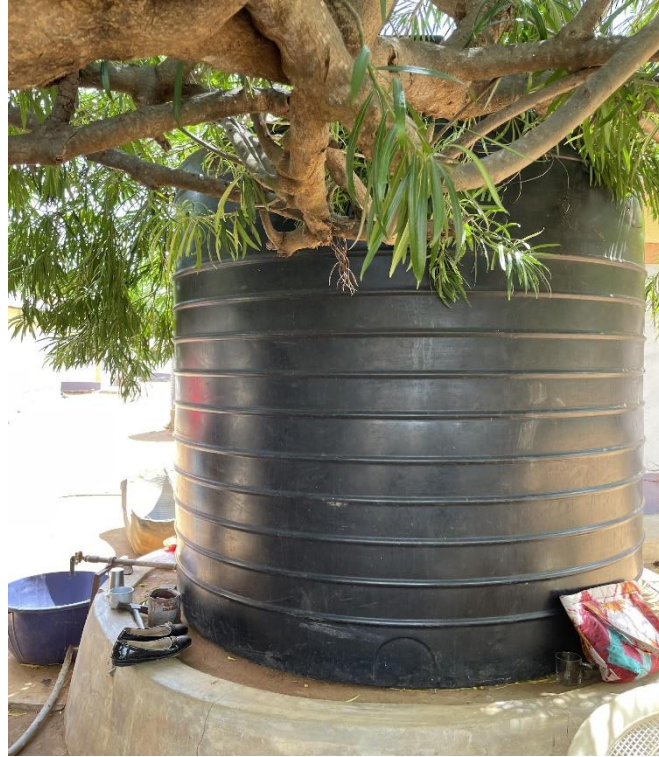
Image 15A: Example of a tank installed under tree shade to help improve life of the storage tank
