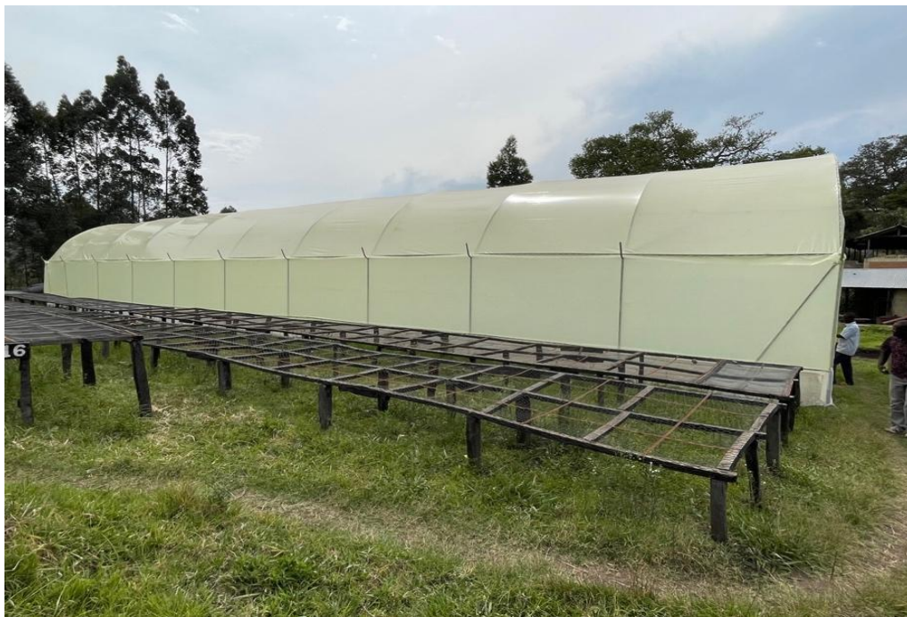
Image 4B: Solar tunnel dryer alongside wooden dryers with rusted wire mesh
