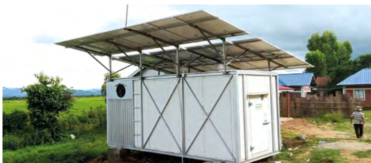
Figure 5.4 Application of solar energy to a cold room ( Infricold ).
