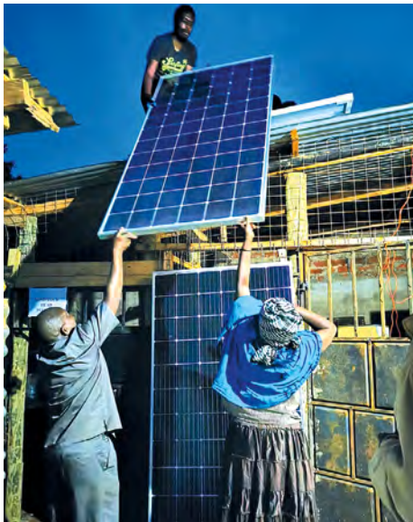
Figure 6.8 PV modules installation ( Solar Cooling Engineering ).
