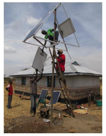
Photo 1 Elaborate and expensive pole mounting for PV SMART systems
