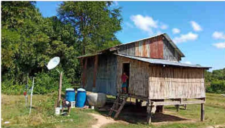
Pom's house, with a small 70W Solar Home System installed on the edge of the lower roof.
