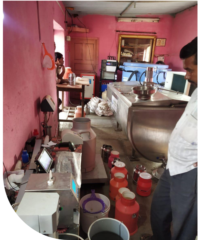
Promethean's milk chilling and remote monitoring technology at a site in Tungi
