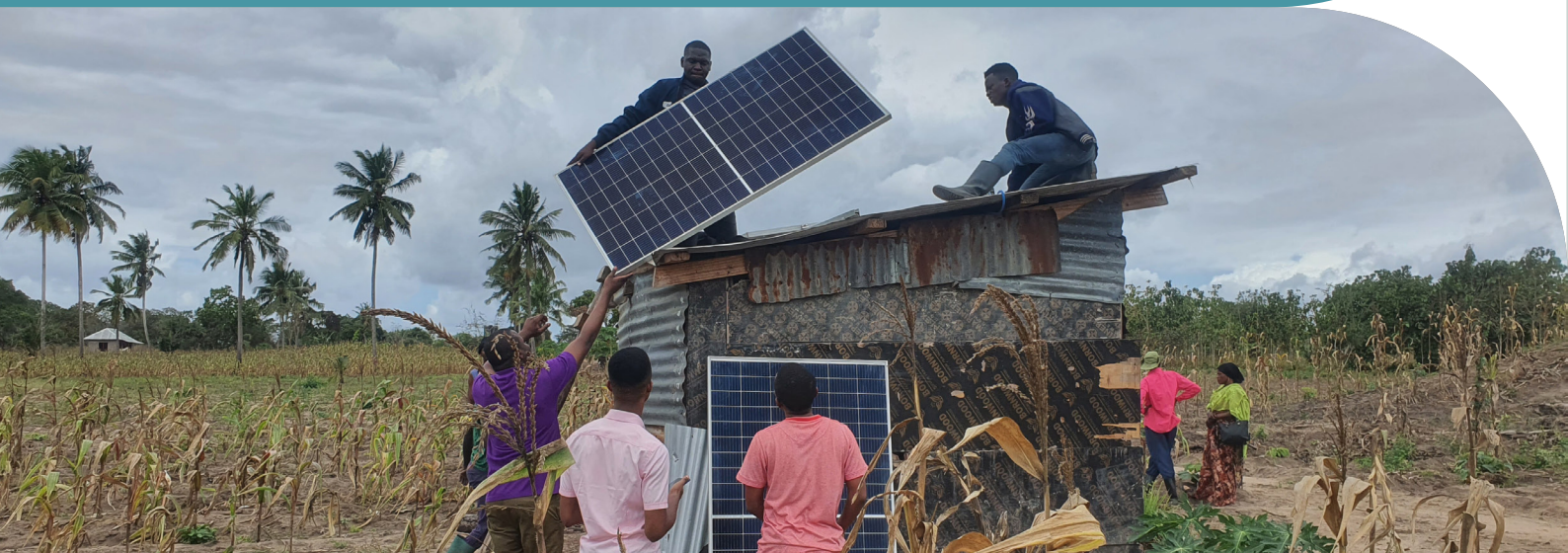
A solar water pump system being installed in Tanzania
