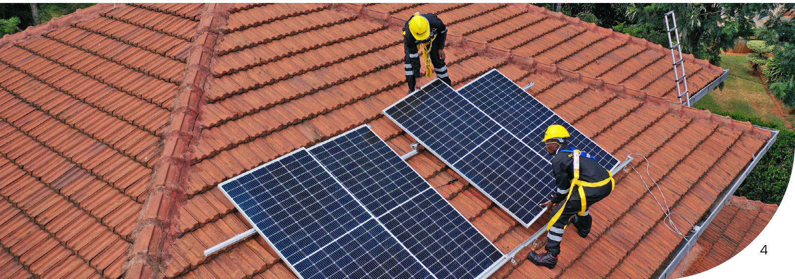
Sun King's engineers installing solar panels
