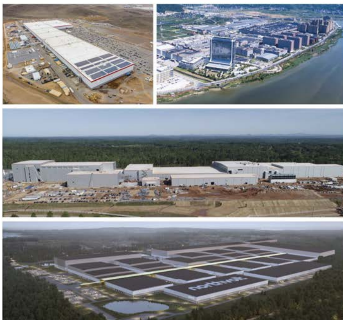
Figure 12. Li-ion factories around the world from clockwise from top left: Tesla's 35 GWh factory in Nevada; CATL's HQ and 45 GWh factory in Ningde, China; SK's 10 GWh factory in Georgia; rendering of Northvolt's 16 GWh facility under construction.
