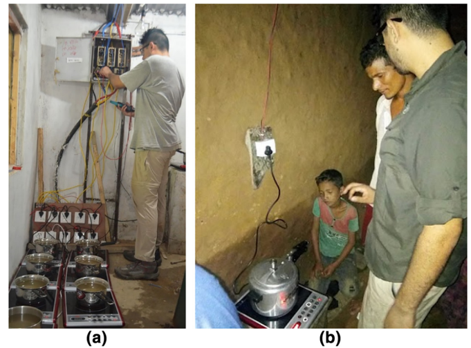
Fig. 3. (a) Testing induction hobs in the MHP powerhouse and (b) user training on cooking with the pressure cookers on the induction hobs.
